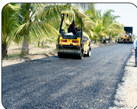
Construction of Farm WBM road
